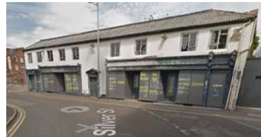
Silver Street. Source: Google Street View 2015
