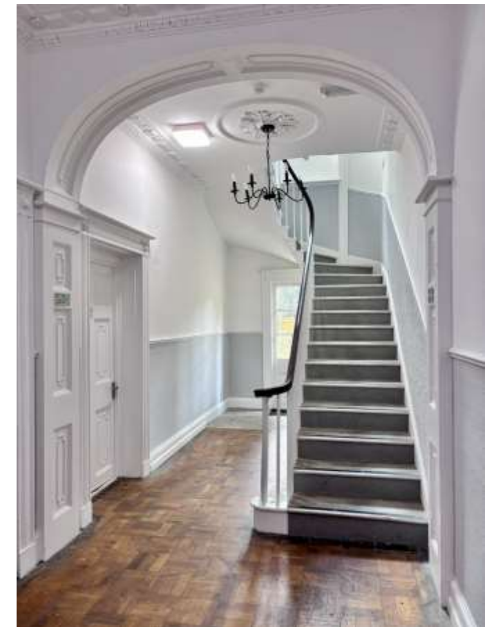
Entrance hall: open-well staircase with winders, wretched handrail, square baluster & modillion plaster cornice
