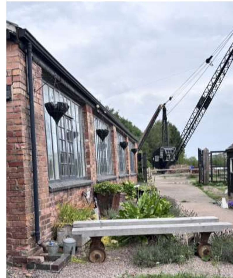
Workshops and restored crane
