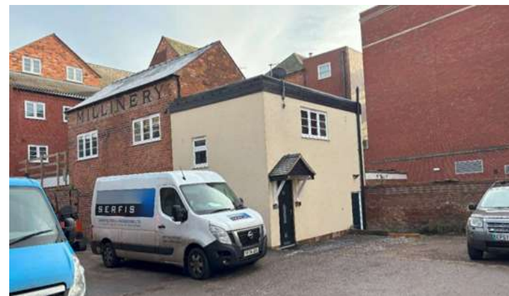
Existing modern extension – the proposals would extend to the right. Source: Masefields
