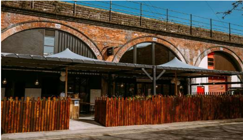
An area missing from the draft SPD – the uniformity of shopfront design to the railway arches. Source: @PershorePatty.
