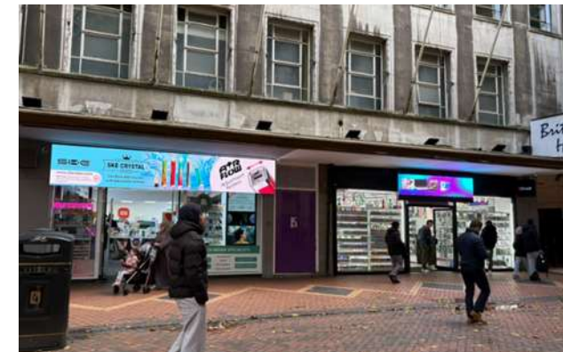
A current proliferation of LED dot matrix moving image signage fascias in Birmingham
